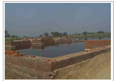
Restoration work at Chandra Sarovar Chaumuha
