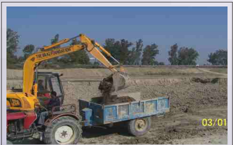
Desilting in process at a Kund
